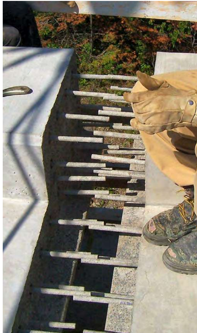
Rainy Lake - 2006, MTO NW Region Pre-cast panels decks
