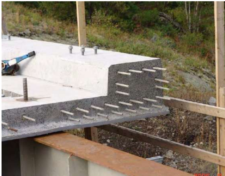
Rainy Lake - 2006, MTO NW Region Pre-cast panels decks
