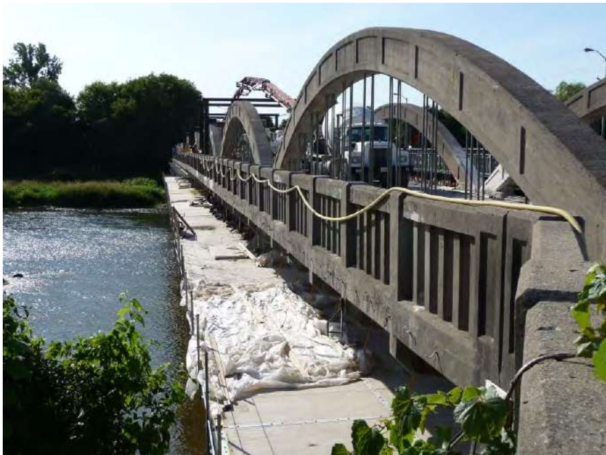
Bridgeport Bridge deck replacement Region of Waterloo, ON
