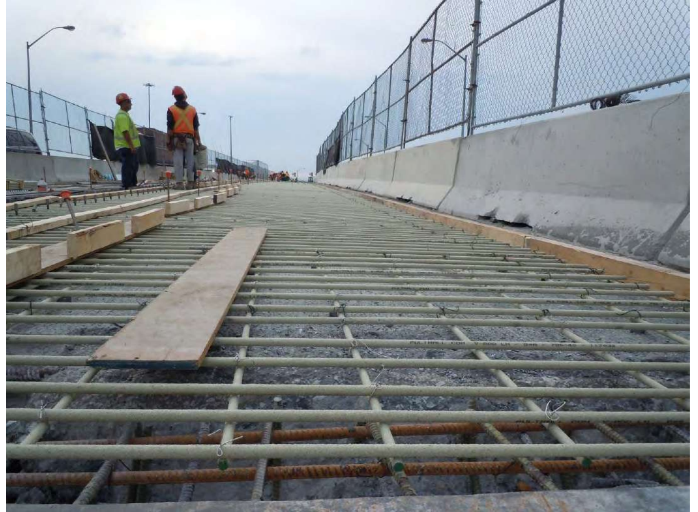
MTO 2010-2054 (Warden Ave over Hwy 401 in Toronto - bar on site and placed in deck
