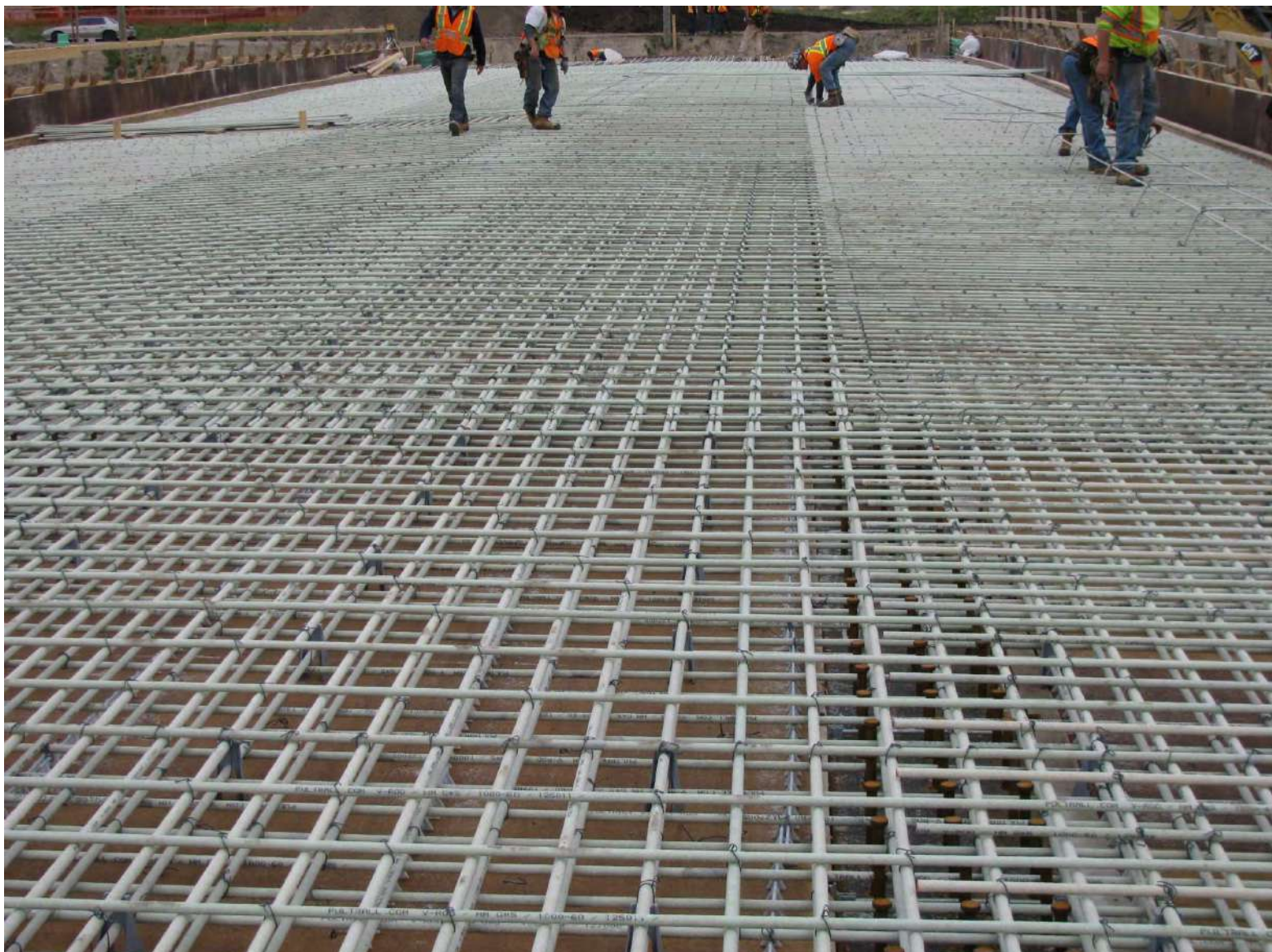
Dorchester Bridge, Kitchener, ON
